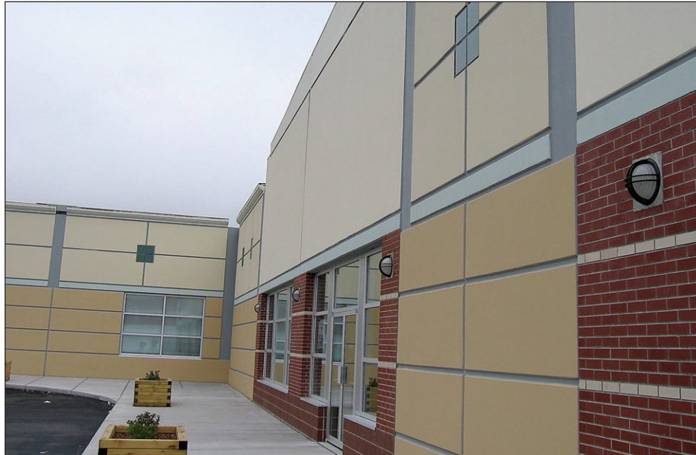
Top: Suited to both tilt-up and precast, the Mbrick system used in the Downsview Mall expansion project is a method of embedding veneer brick in concrete to create the appearance of masonry.
