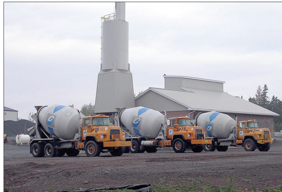
Casey Concrete Ltd. opened a new plant this past summer in Antigonish, N.S. The Stephens LT9 plant and batching system by BMH Systems Inc. is capable of producing 175 cubic metres per hour. Headquartered in Truro, N.S., Casey's owns and operates two ready mix plants in New Brunswick and five plants in northern Nova Scotia.
