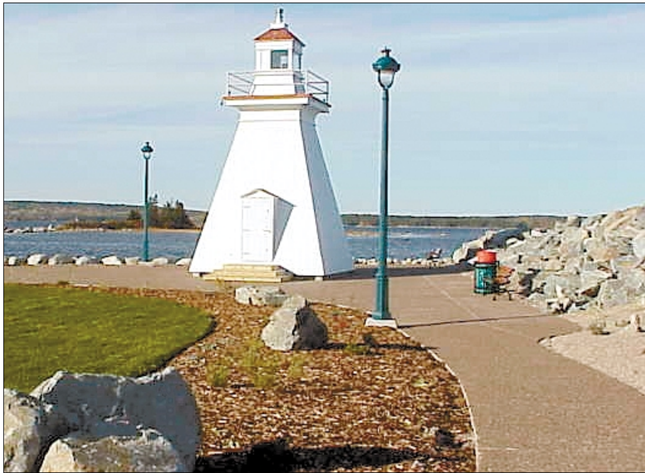
The Port Medway Lighthouse Park in Queens County, NS was completed in Fall 2002 to showcase this historical 1899 lighthouse. South Shore Ready Mix Limited supplied the exposed aggregate concrete for over 1200 m 2 of walkways in the park.
