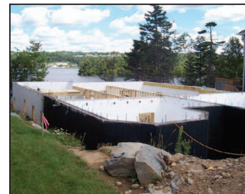
Mike Perrier, Perrier's Concrete Homes, Dartmouth, N.S. is one of few residential contractors in Atlantic Canada who builds exclusively with insulating concrete forms (ICF). Mike and his all-deaf crew have become specialized with the IntegraSpec® ICF wall system over the past five years, raising the building envelope only. This beautiful single-storey home, built last summer, overlooks Lake Banook in Dartmouth.
