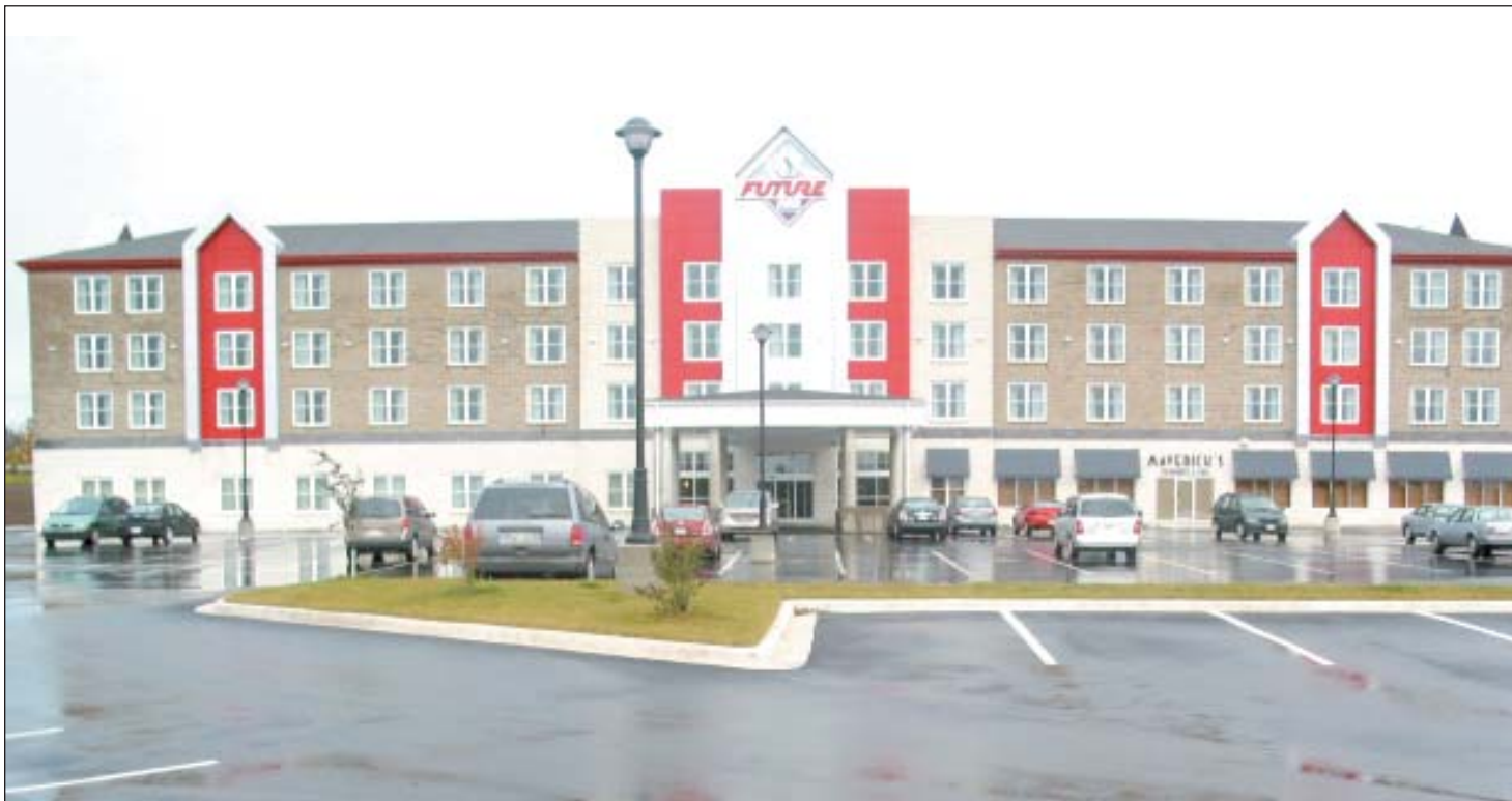
The Future Inns in Moncton chose the NuDura ICF Wall System, supplied by Bird-Stairs Limited, to build a four-storey hotel that opened in the spring of 2006. The project is owned by Future Inns; the architect was Anderson Architect Ltd. of Halifax; the structural engineer was Pinto Engineering Ltd. of Halifax; the project superintendent was Tri-Cor Development; the project manager was Steven Campbell; the NuDura ICF system supplier was Neil Reid of Bird Stairs Limited of Moncton; the NuDura ICF system installer was Ken Allen of Braemar Management Inc. of Salisbury; and the ready mixed concrete supplier was Casey Concrete Limited of Moncton.
