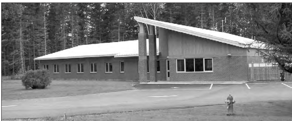
The Department of Natural Resources office in Bathurst, N.B. was completed in 2005 and is rated LEED Silver. It's a 585 square metre ICF building, built substantially in winter, with some exterior walls over seven metres high. The architect was Pam Barteaux of the N.B. Department of Supply and Services; the structural engineer was Larry MacLaggan of Miramichi Engineering Ltd.; the general contractor was Stephane McGraw of Gloucester Construction Ltd.; the Eco-Block ICF system supplier was John Landry of Arrow Construction Products Limited; and the ready mixed concrete supplier was Blanchard Ready Mix Ltd. of Dunlop, N.B.
