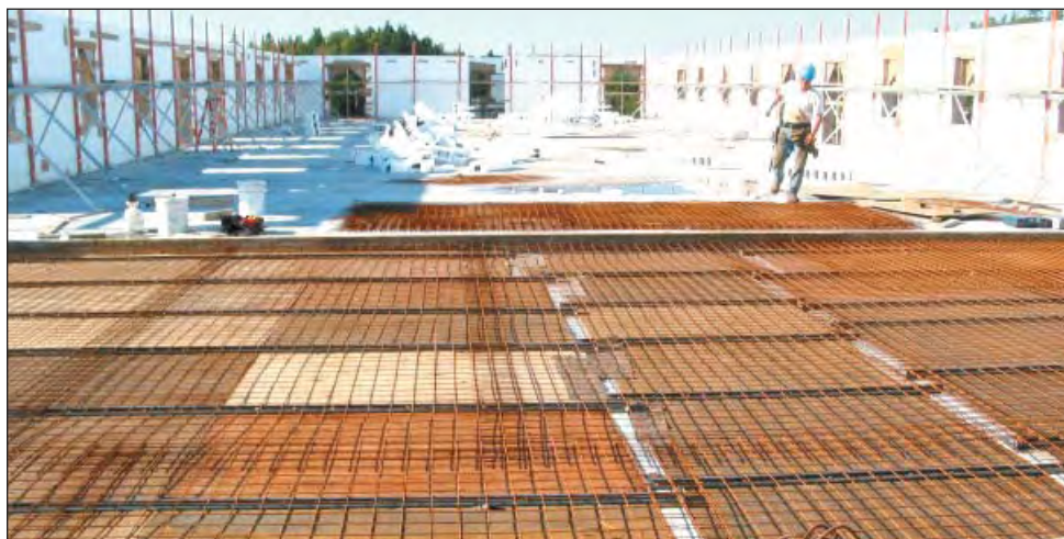
This three-story, 60-unit ICF apartment building in Saint John, N.B. is nearing completion. Fern-Co Building Concept Inc. of Rogersville, N.B., the project's owner-developer, did the job with its own forces, using the Hambro floor system and the AMVIC Building System for the exterior walls. Residents, mostly seniors and retirees, will enjoy the benefits of quiet and warm, energy efficient living spaces. Concrete was pumped (in part) by AMVIC distributor, MacLeod General Construction Ltd., Centreville, N.B. and supplied by Lafarge Aggregates, Concrete and Asphalt from its nearby plant.
