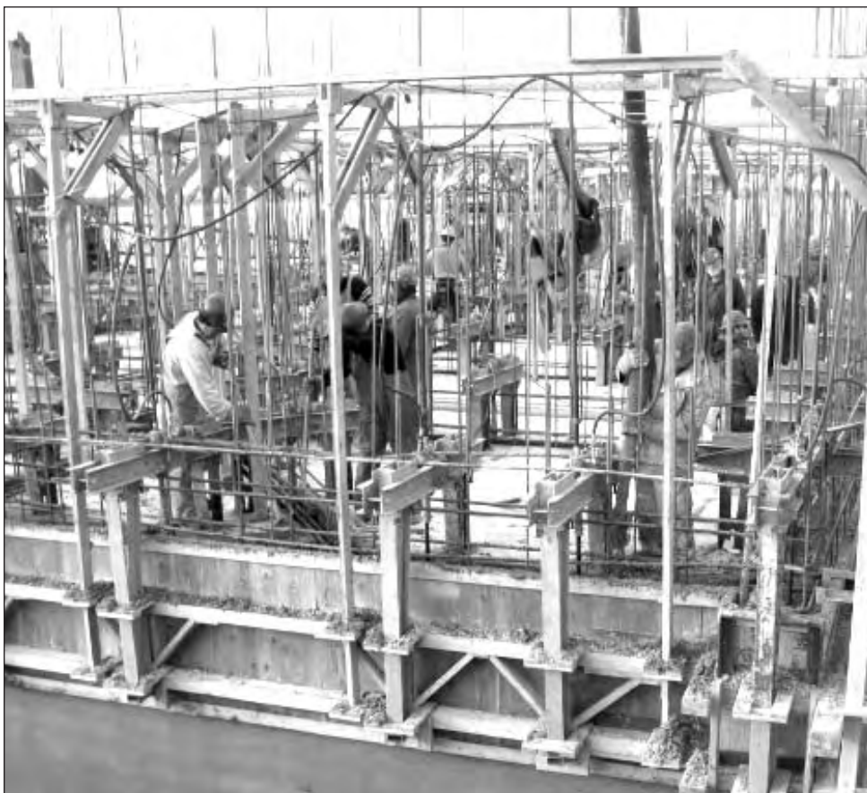
The Charlottetown Harbour Authority is expanding the city's Marine Terminal Wharf near the historic downtown. The project, scheduled to open in August 2007, required the construction and sinking of five floating concrete cribs, each measuring 35m x 14m x 15m high. The contractor is Beaver Marine Inc. Schurman Concrete Limited of Charlottetown, which will supply 11,000 cubic metres of concrete by the time the project is complete, including several continuous pours of eight, 12 and 24 hours duration.
