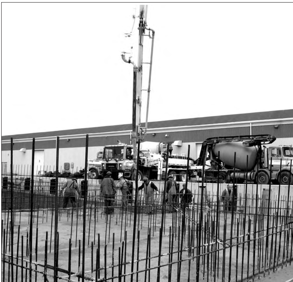
The Charlottetown Harbour Authority is expanding the city's Marine Terminal Wharf near the historic downtown. The project, scheduled to open in August 2007, required the construction and sinking of five floating concrete cribs, each measuring 35m x 14m x 15m high. The contractor is Beaver Marine Inc. Schurman Concrete Limited of Charlottetown, which will supply 11,000 cubic metres of concrete by the time the project is complete, including several continuous pours of eight, 12 and 24 hours duration.
