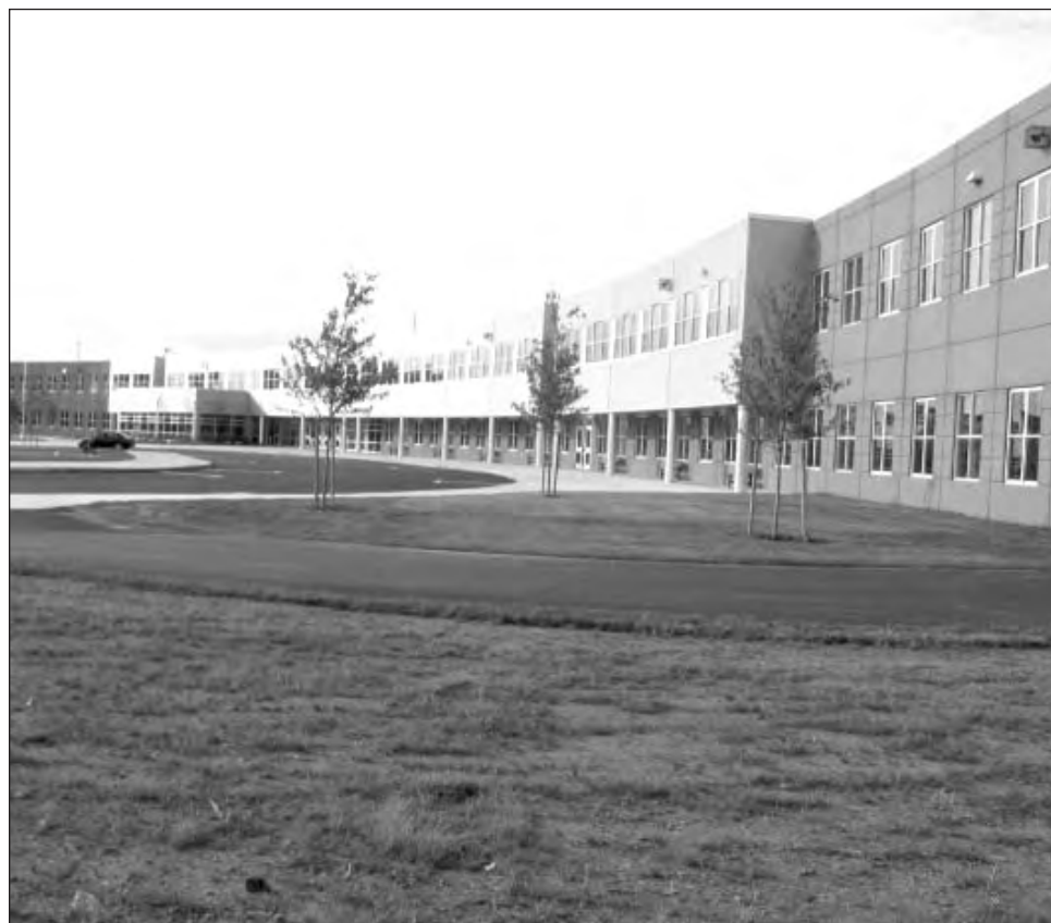
The new Sir John A. MacDonald High School was completed in less than one year using the tilt-up method, and opened on schedule for the start of school in September. Rideau Construction Inc. of Bedford, N.S. built the project, including the tilt-up walls. Quality Concrete of Dartmouth, N.S. supplied the concrete.
